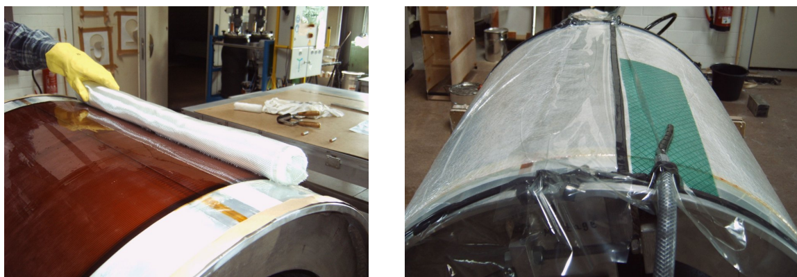
(a) application of the GRP
