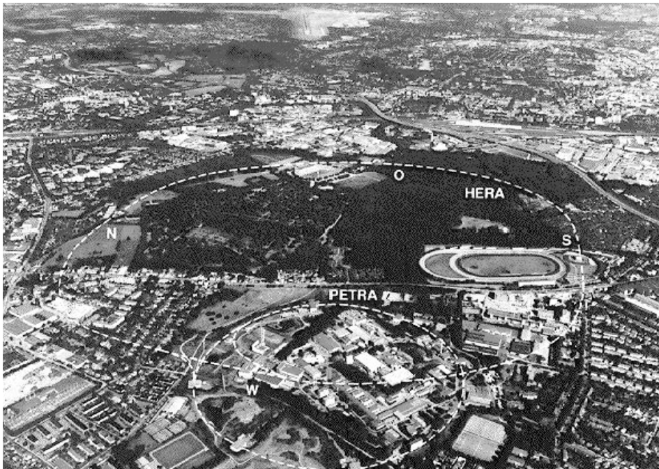
Fig. 3.1 View of DESY from an aeroplane approaching Hamburg airport from the west [85]. The location of the HERA and PETRA storage rings is indicated by the dashed outlines. While most of the other DESY buildings are encircled by the PETRA ring, the HERA south hall with the ZEUS detector is situated off the DESY main ground at the place marked with S, right beside the trotting course.
