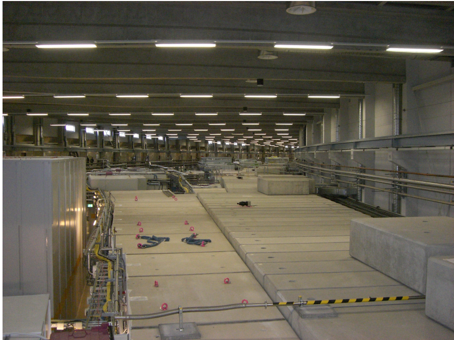
(a) View along the storage ring: On the right runs the storage ring, on the left beamlines are attached tangentially.
