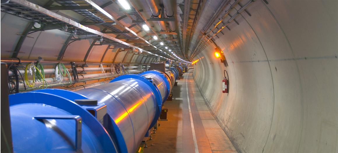
Figure 2.1.: A view from inside one of the arcs of the LHC accelerator tunnel: the blue cylinders in the foreground are the superconducting dipoles used to steer the protons into a circular orbit. Image from [54].
