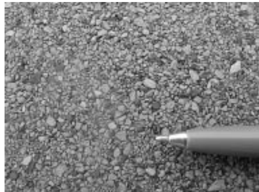
Green roof paper (close-up)
